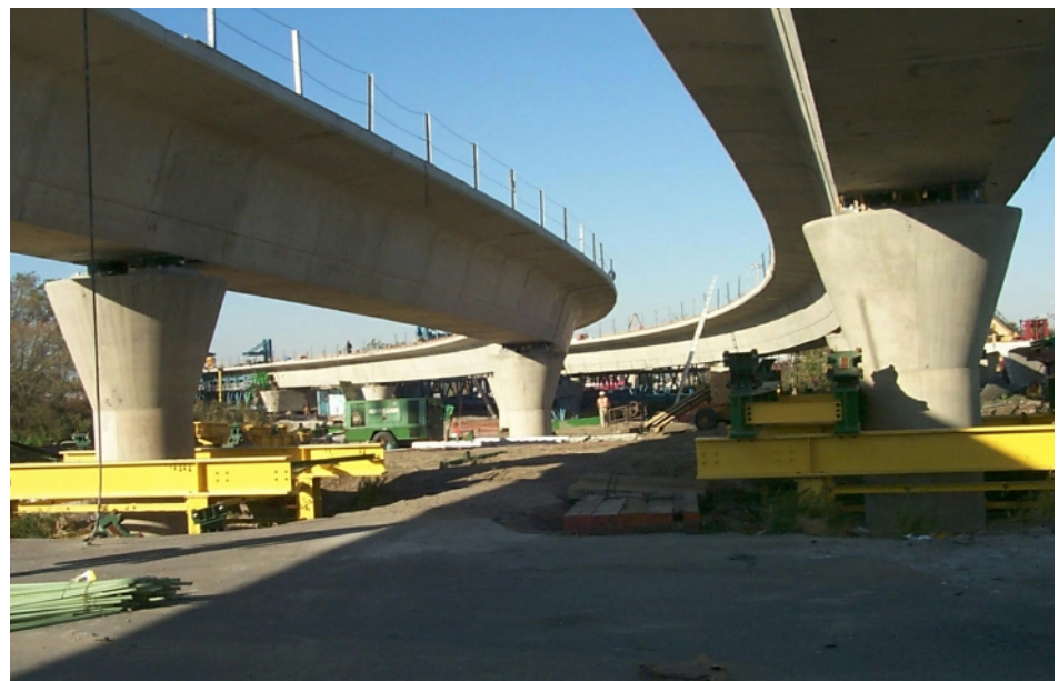
Erected guideway at Howard Beach Wetlands section.
