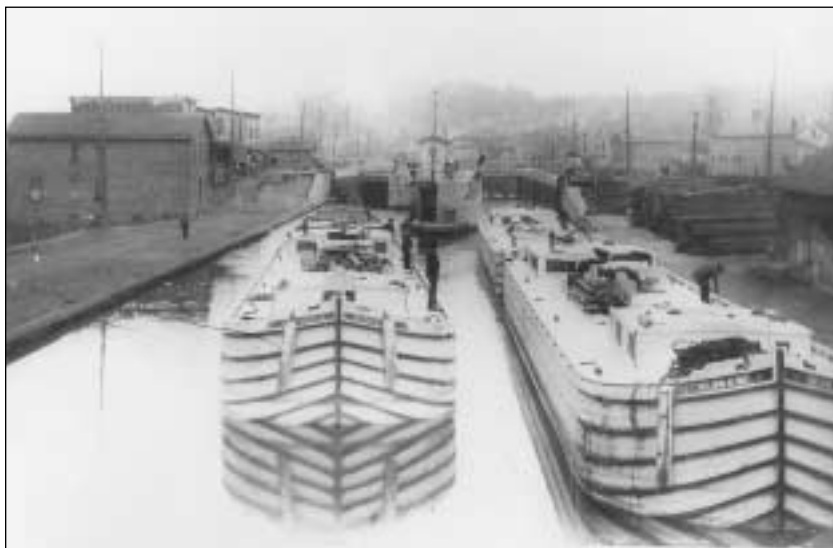
Double locks at Beech Street, Syracuse, New York, date back to 1835 enlargement of canal (circa 1900).
