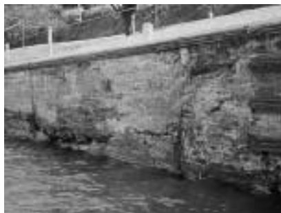
Deteriorated wall at Monongahela River Lock and Dam 3, which opened in 1907.
