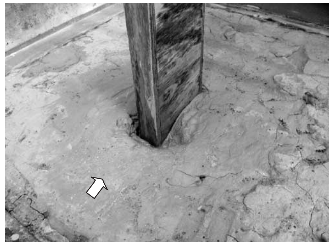
Figure A12 Scour Hole in Test Sh-3.
