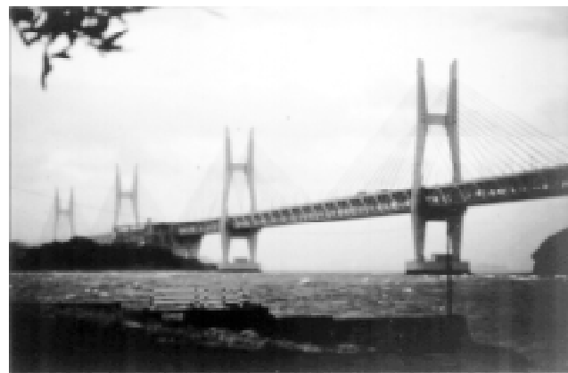
Figure 1. Cable-stayed bridges on the Kojima-Sakaide Route.
