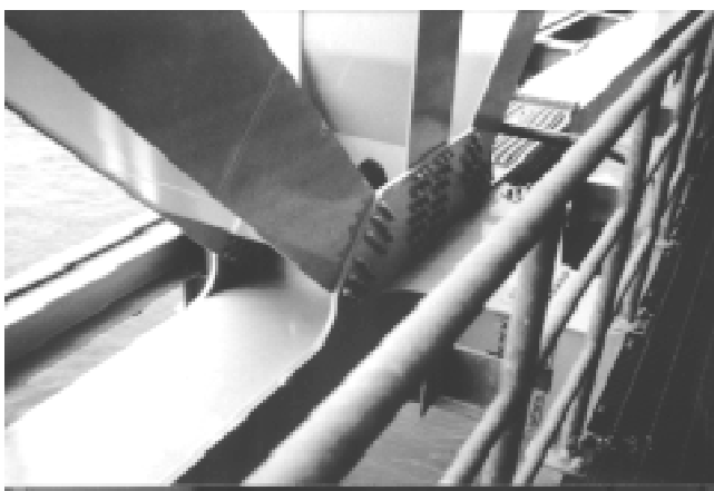
Figure 28. End connection of tapered members.
