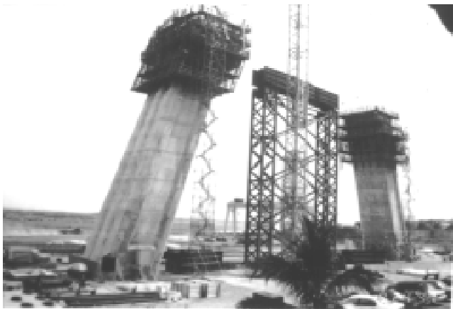
Figure 13. Kao-Ping River Bridge under construction.
