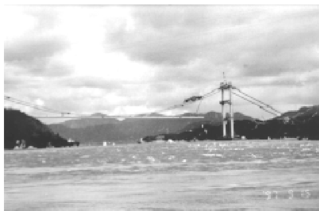
Figure 6. Kurushima 1 under construction.
