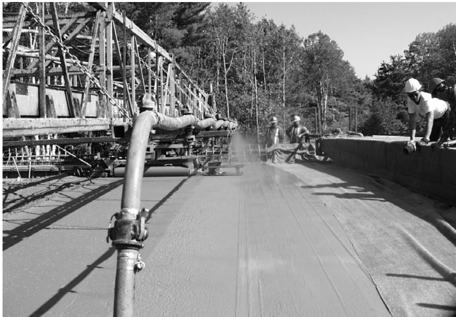
FIGURE 6 Application of wet burlap immediately after concrete curing (Schell and Konecny 2001). (Courtesy: HPC Bridge Views published by FHWA and NCBC.)
