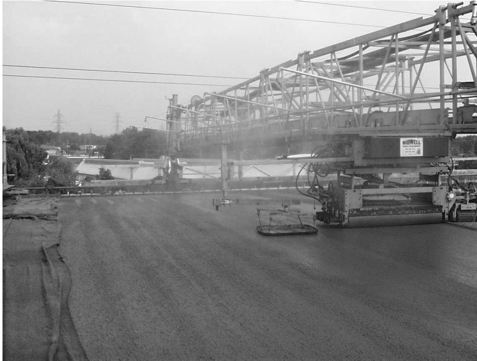
FIGURE 7 Nozzles attached to the finishing equipment (Schell and Konecny 2001). (Courtesy: HPC Bridge Views published by FHWA and NCBC.)
