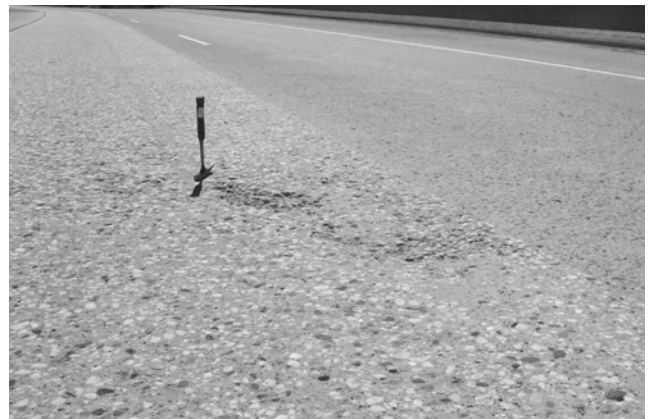
FIGURE 3 Abrasion damage caused by chain wear.
