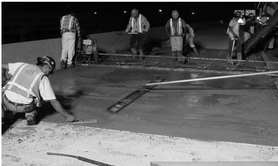
FIGURE 4 Placement of a latex-modified overlay.
