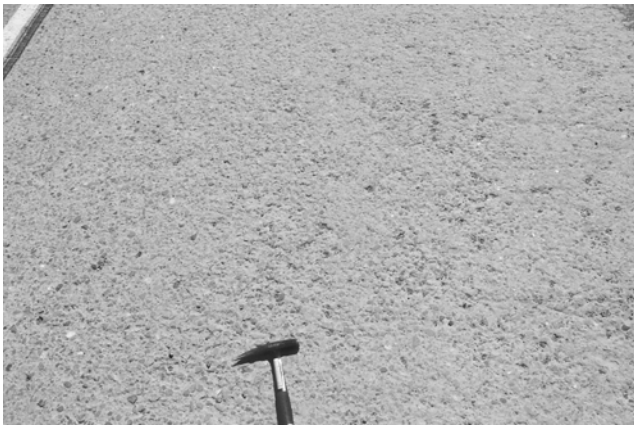
FIGURE 1 Surface scaling caused by freeze-thaw cycles.
