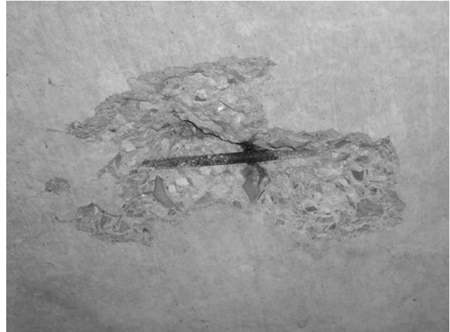
FIGURE 2 Spalling caused by corroded reinforcement.
