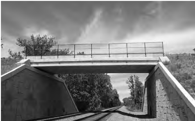
FIGURE 1 Single-span box beam bridge over railroad (Source: New York State DOT).
