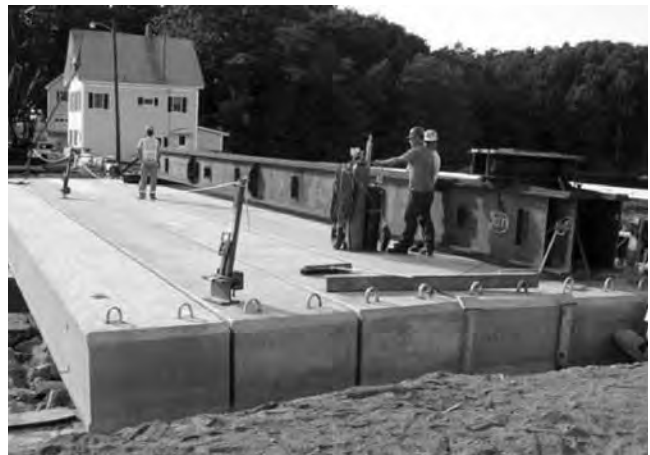
FIGURE 4 Adjacent box beams used for the superstructure of the Davis Narrows Bridge, Maine (Source: Maine DOT).
