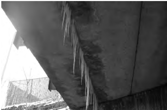
FIGURE 20 Leakage through longitudinal joints (Source: Pennsylvania DOT).
