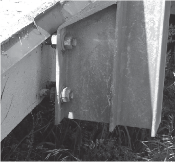
b. Steel barrier
