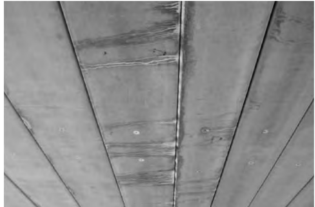
FIGURE 21 Efflorescence on the underside, indicating leakage through the joints (Source: New York State DOT).
