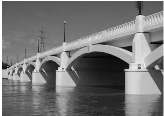
FIGURE 3 Adjacent box beam bridge to replicate an arch bridge (Source: Henry G. Russell).
