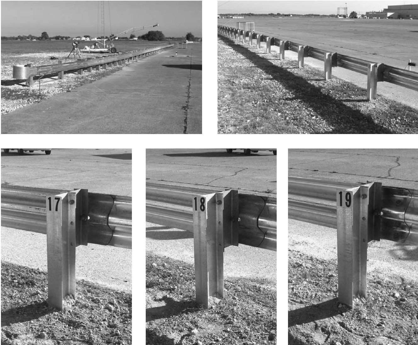
Figure 30. G4(1S) guardrail installation before test 472480-1.
