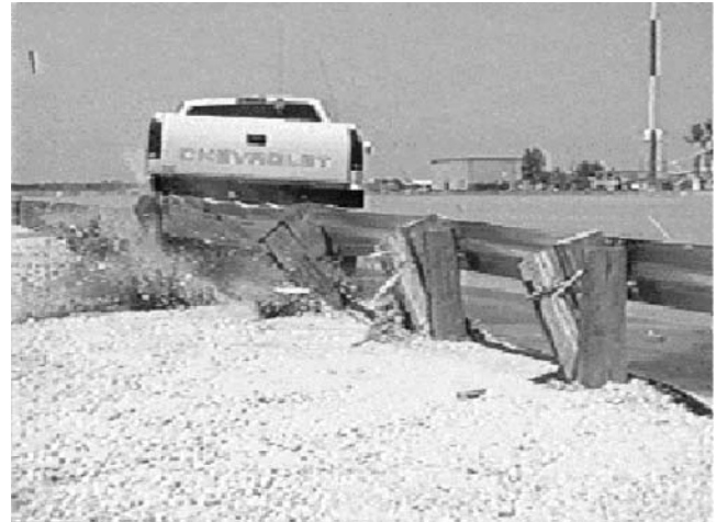
Figure 11. Guardrail damage in TTI Test 404201-1.
