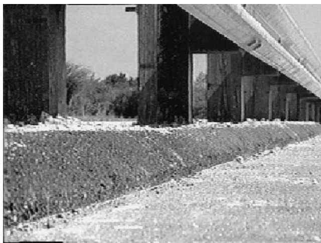
Figure 10. Guardrail-curb installation for TTI test 404201-1.
