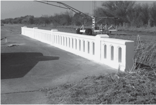
Figure 42. Texas T411 aesthetic bridge rail.
