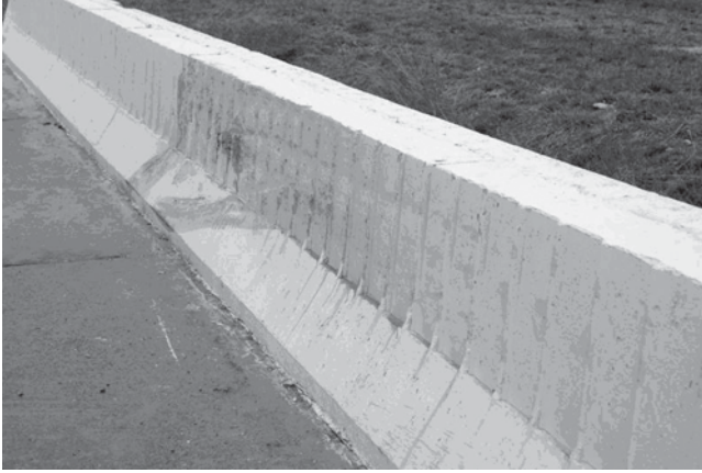
Figure 70. Barrier damage for Crash Test 2.
