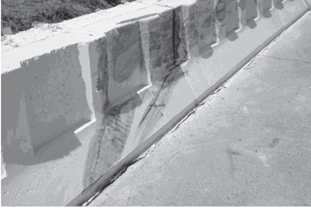
Figure 81. Barrier damage for Crash Test 7.
