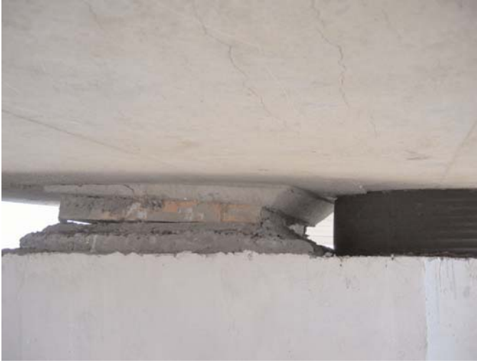
Figure 2-1. Uplift at edge of bearing.
