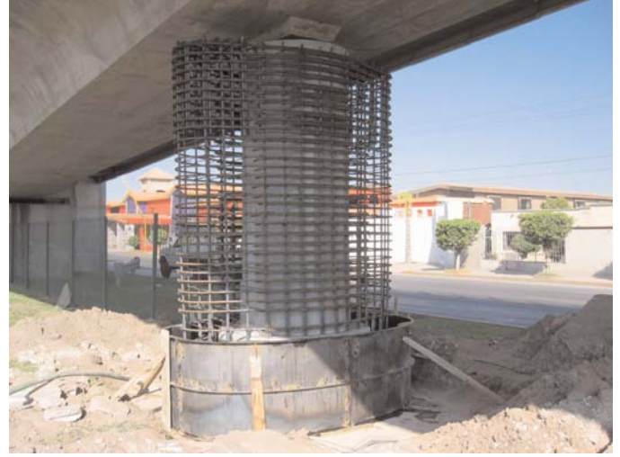
Figure 2-2. Construction of widened column.
