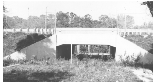
FIGURE 24 Box culvert underpass used on SR-29 in southern Florida.
