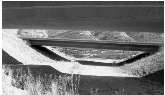
FIGURE 9 Bridge overdry wash used by wildlife on Highway 58 in California.
