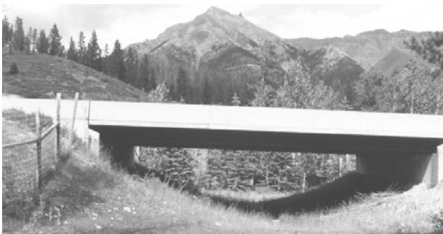
FIGURE 26 Underpass in Banff National Park, Alberta.
