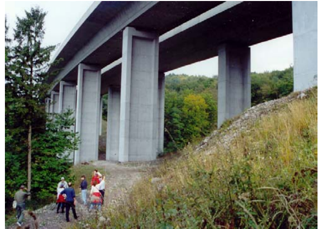
FIGURE 18 Viaduct on the Ljubljana–Trieste Highway in Slovenia.
