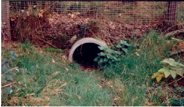
FIGURE 1 Fine mesh fence and culvert for small mammals in Europe.
