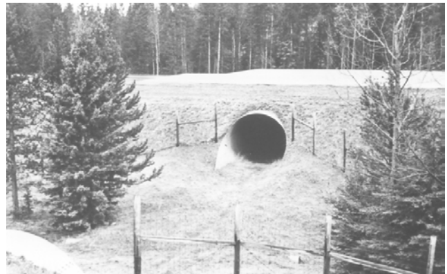
FIGURE 16 Large pipe culvert being used by a variety of wildlife in Banff National Park, Alberta.
