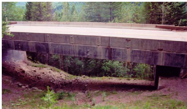
FIGURE 10 Goat bridge underpass on Highway 2 near Glacier National Park.
