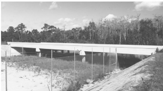
FIGURE 23 One of 23 wildlife underpasses on I-75 (Alligator Alley) in southern Florida.
