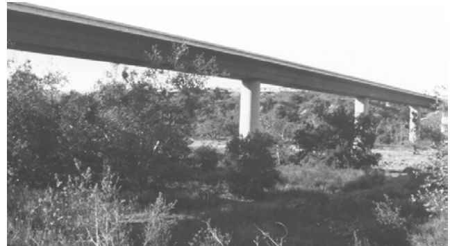
FIGURE 19 Viaduct on Highway 241 in southern California.
