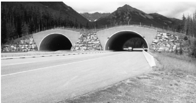
FIGURE 25 Large overpass used by wildlife in Banff National Park, Alberta.
