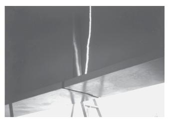
FIGURE 17 View of cracked girder in two-girder span of I-79 Bridge at Neville Island in Pittsburgh as an example of a two-girder bridge that is sufficiently redundant to avoid collapse despite a fracture of the tension flange and the web of one girder.
