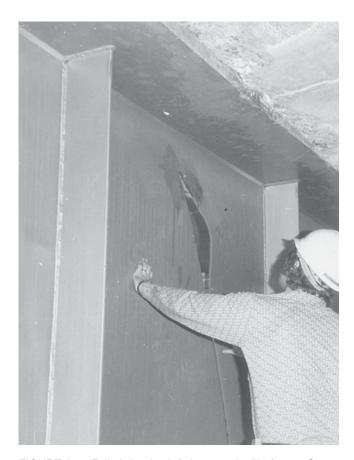
FIGURE A12 Full-girder-depth fatigue crack of Lafayette Street Bridge in St. Paul, Minnesota.
