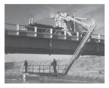
FIGURE 5 Snooper used for hands-on inspection from bridge deck.
