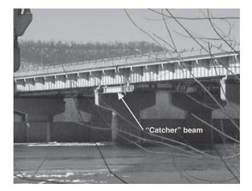
FIGURE A16 Catcher system as used on a typical pin and hanger bridge. (*Courtesy:* Modjeski and Masters, Inc.)
