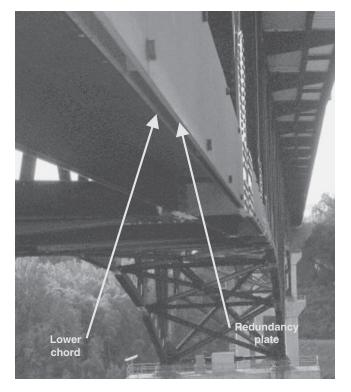
FIGURE 13 Redundancy plate bolted to lower chord of SR-33 bridge near Easton, Pennsylvania. (*Courtesy:* HNTB.)
