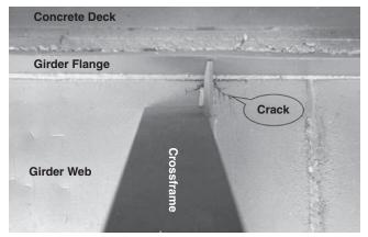
FIGURE 3 Typical web-gap fatigue cracking.
