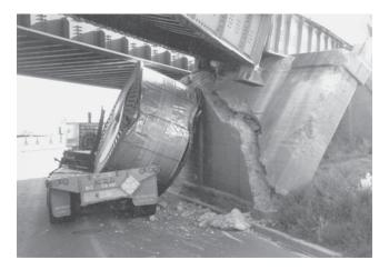
FIGURE 7 Example of vehicle–bridge collision causing collapse owing to nonredundant substructure. (*Courtesy:* Robert Sweeney.)
