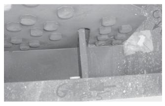
FIGURE A3 Fractured girder of the Hoan Bridge in Milwaukee (top) and view of critical shelf plate detail featuring intersecting welds.
