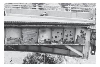
FIGURE 4 Collapse of Mianus River Bridge. (*Courtesy:* John W. Fisher.)
