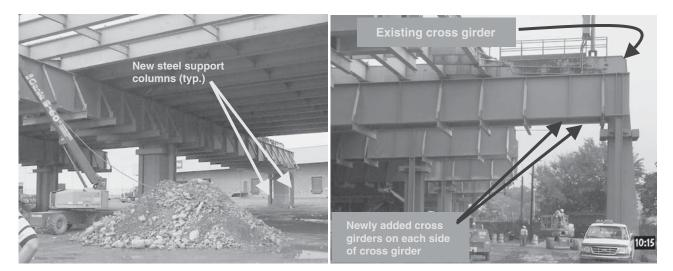
FIGURE A15 Additional support girders are used to provide redundancy to steel cross girders on I-95 bridge north of Philadelphia, Pennsylvania.
