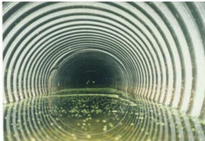
Figure 2 – An interior view of the pipe from outlet end
