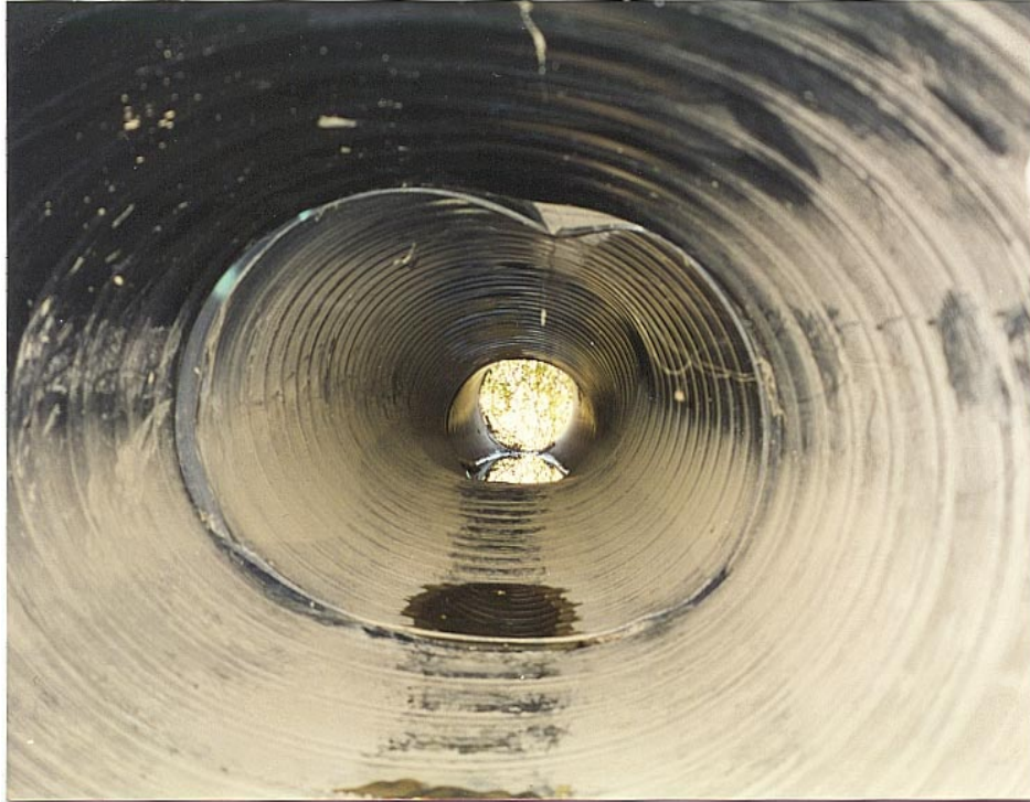
Figure 1 – An interior view of the pipe at Site R
