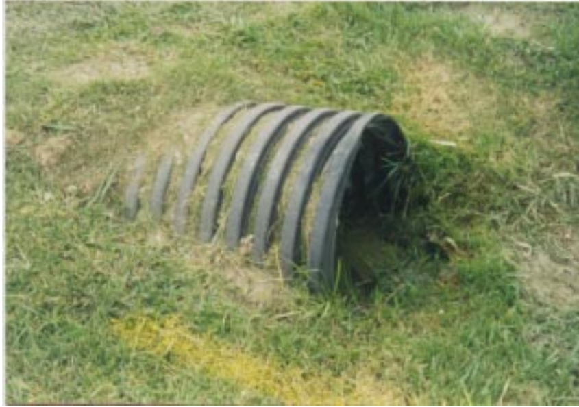
Figure 1 – A general view on the pipe at Site N
