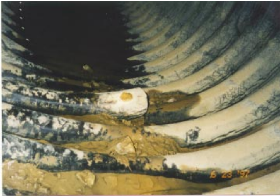
Figure 1 – An interior view of the pipe in Site A
