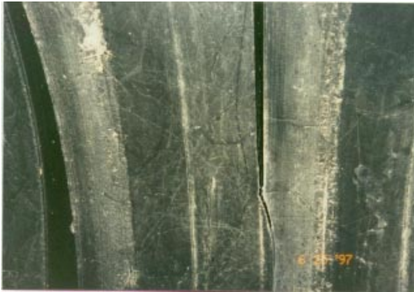
Figure 2 – Long circumferential crack in Sample H2
