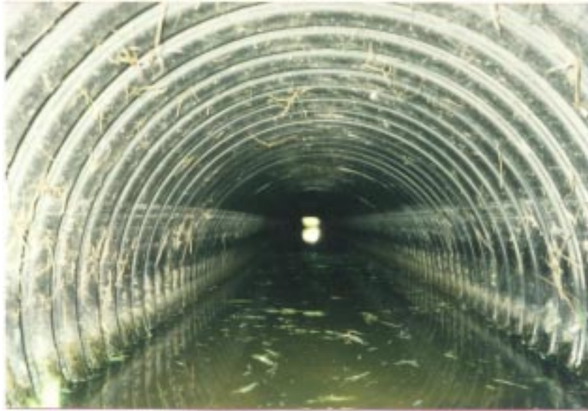
Figure 2 – An interior view of the pipe from the outlet end
