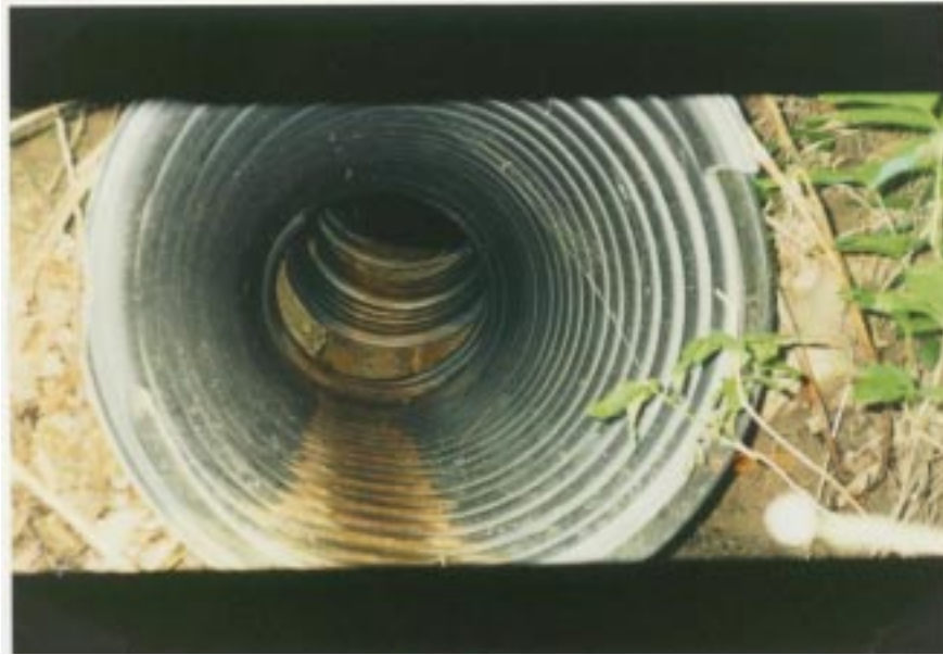
Figure 1 – General view of the pipe in Site B
