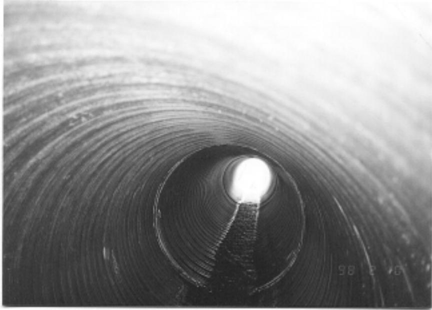
Figure 1 – An interior view of the pipe at Site W
