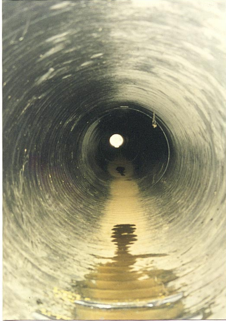
Figure 1 – An interior view on the pipe at Site P
