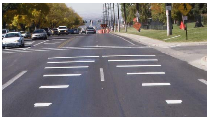
Figure D-7. Five-Bar Triangle Advance Crosswalk Pavement Markings in Salt Lake City, Utah. (Source: Tim Harpst, Salt Lake City, Utah, U.S.A.)
