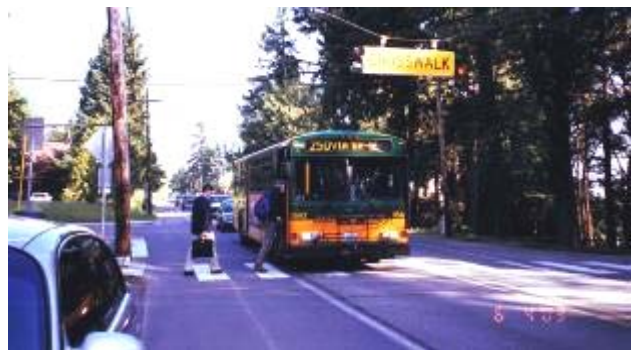
(b) Marked Crosswalk
