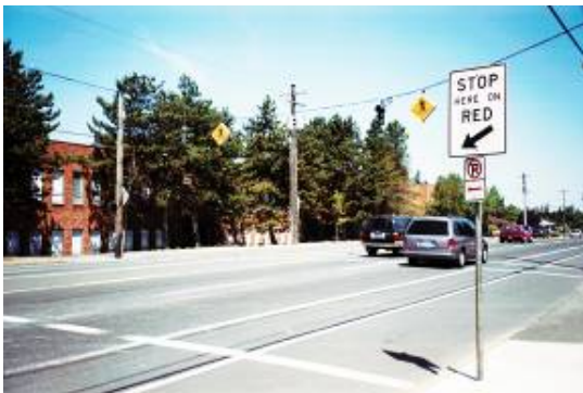
(a) Pedestrian Signal with Advance Stop Bar
