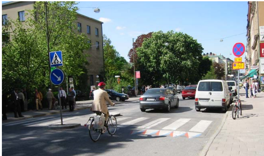
Figure D-17. Painted Raised Crosswalk in Stockholm, Sweden.
