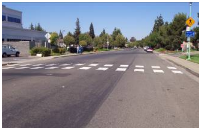
Figure D-6. Triple-Four High-Visibility Markings in Sacramento, California. (Source: Nazir Lalani, Ventura County, California, U.S.A.)
