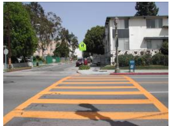
(c) Marked Crosswalk near a School
