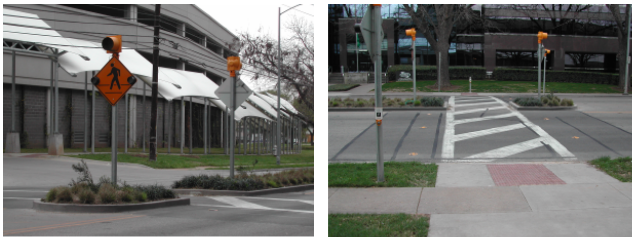
Figure K-2. In-Roadway Warning Lights Treatment at Site 3.
