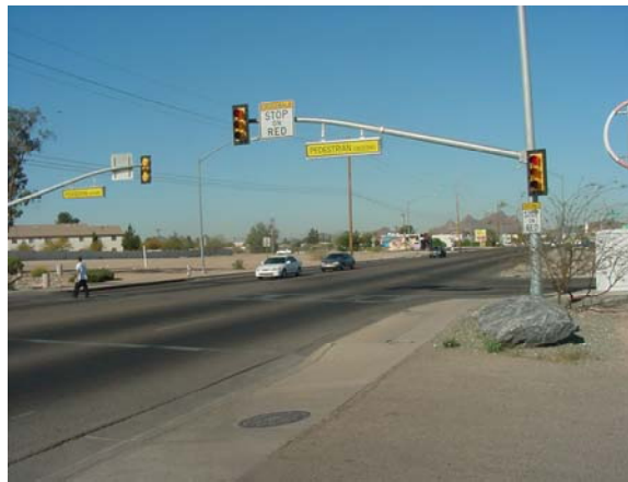
Figure K-3. HAWK Treatment at Site 4.
