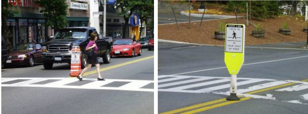
Figure D-15. In-Roadway Signs at Crosswalks in New York State. (Source: James Ercolano, Albany, New York, U.S.A.)
