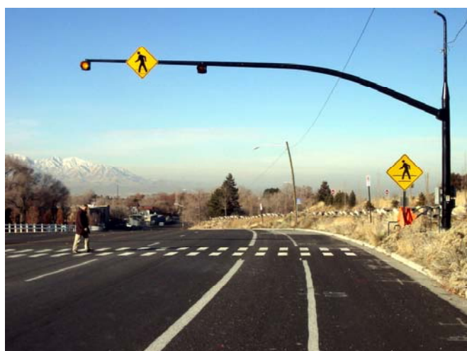
Figure D-4. Pedestrian-Activated Flashing Beacons in Salt Lake City, Utah. (Source: Tim Harpst, Salt Lake City, Utah, U.S.A.)
