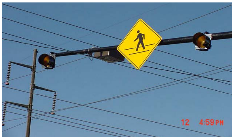
Figure D-5. Pedestrian-Activated Beacons with Light Illumination in Salt Lake City, Utah. (Source: Tim Harpst, Salt Lake City, Utah, U.S.A.)
