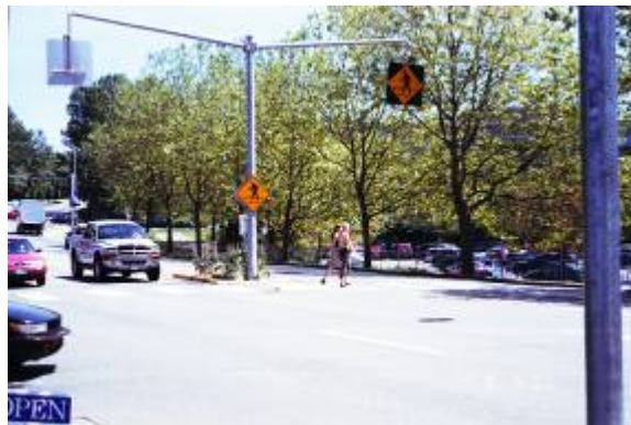
(c) Overhead Signs, Pedestrian Refuge Island at Marked Crosswalk Figure J-4. Example of Treatments in Kirkland.
