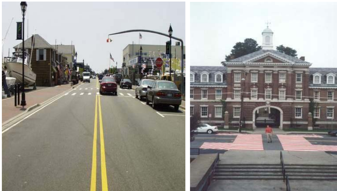
Figure D-14. Crosswalk with Double Piano Style Markings in New York State. (Source: James Ercolano, Albany, New York, U.S.A.)
