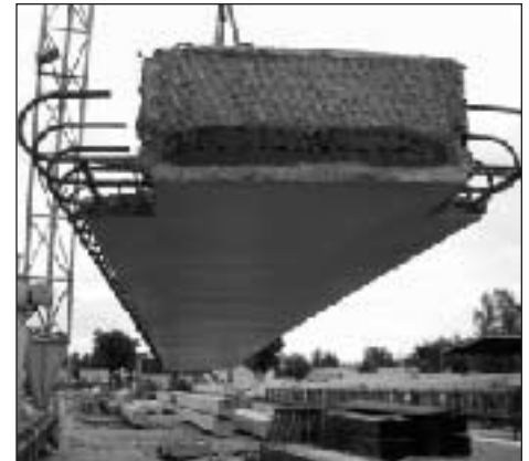
The French Poutre Dalle system eliminates the need for formwork in bridge construction.
