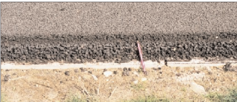
Double Porous Asphalt Pavement Netherlands Roads to the Future
