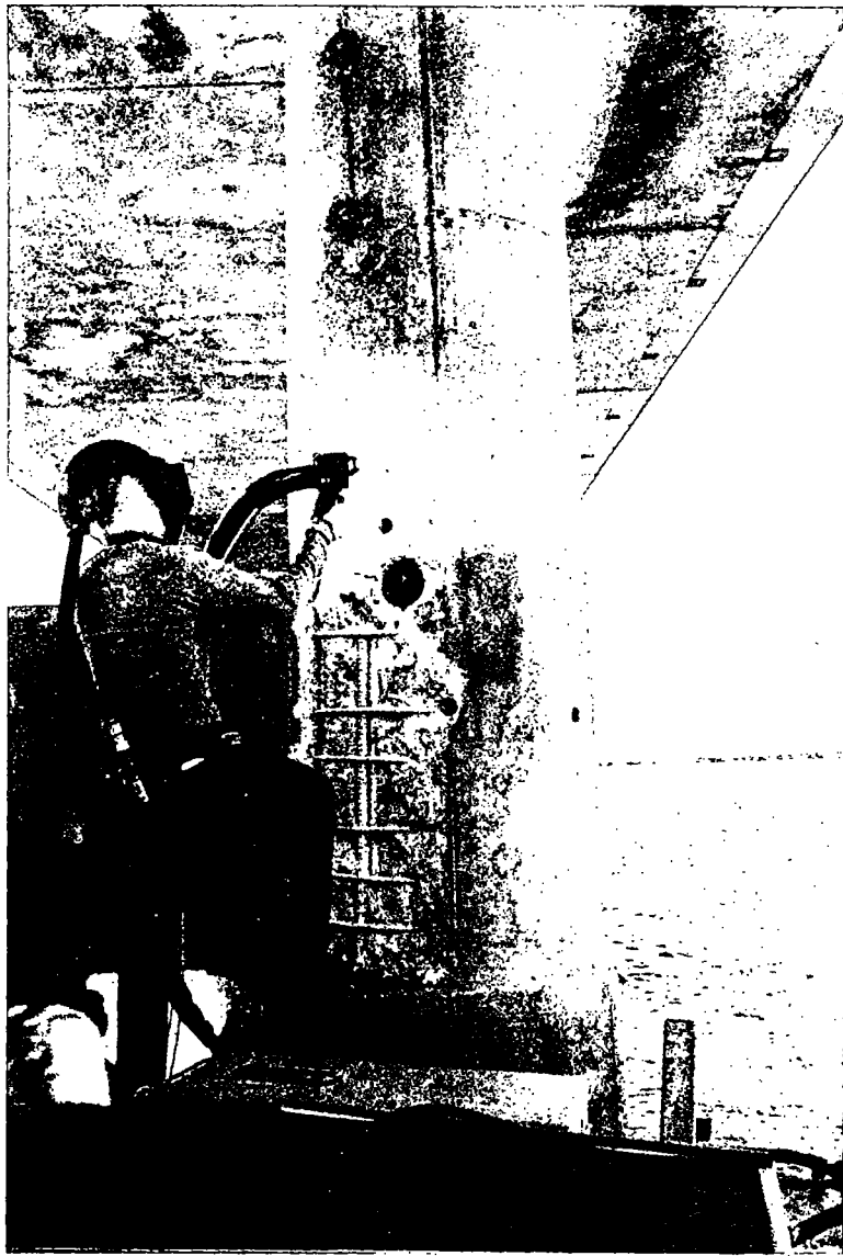
Figure 41. Application of Anode on Reinforcing Steel
