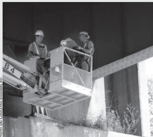
Bridge deterioration is captured on digital photography during inspection process.
