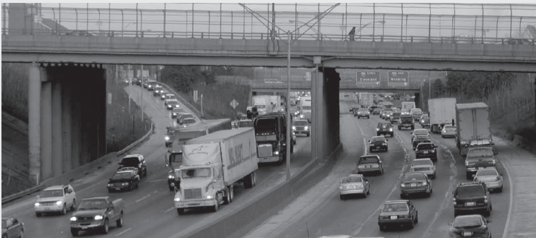
Truck traffic on Ohio highways has grown dramatically over the last 25 years and is expected to increase in the next 20 years. Ohio DOT is addressing the short- and long-term issues of freight transportation by participating in a six-state Upper Midwest Freight Corridor Study that seeks solutions through multistate, multijurisdictional, public-private partnerships.
