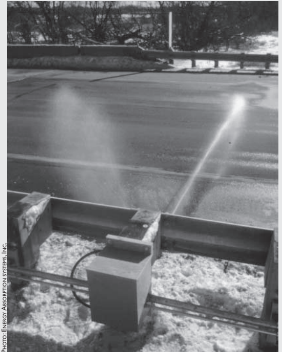
Total storm management techniques for winter services include bridge anti-icing systems.
