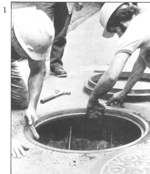
Figure 3. Seating extension ring on the manhole.
