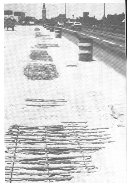
Repairing a concrete bridge deck damaged by corroding reinforcing steel.
