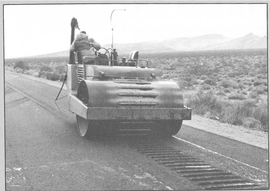
Roller used in California desert project to impress grooves on paved shoulder to alert dozing drivers drifting off highway. (photograph from California Department of Transportation)
