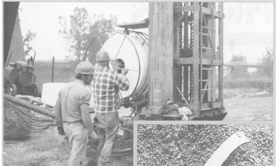
Wick drain on spool for installation.
