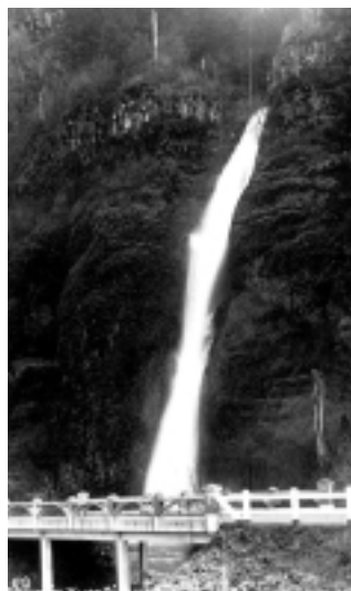
FIGURE 1 Historic Horsetail Falls Bridge, circa 1914.
