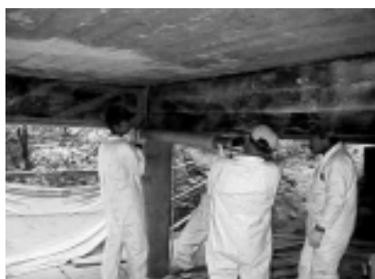
FIGURE 2 Installation of carbon-epoxy sheets on bridge beams.
