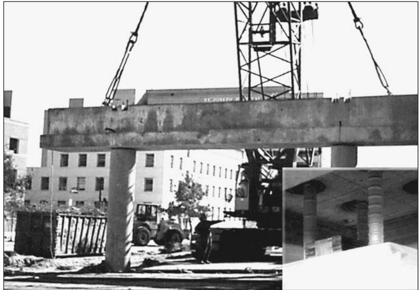
TxDOT's \$18 million research program in 1999. The use of precast bent caps resulted in faster construction and reduced user costs; there is no way to determine exact construction cost savings because construction costs are project specific.
