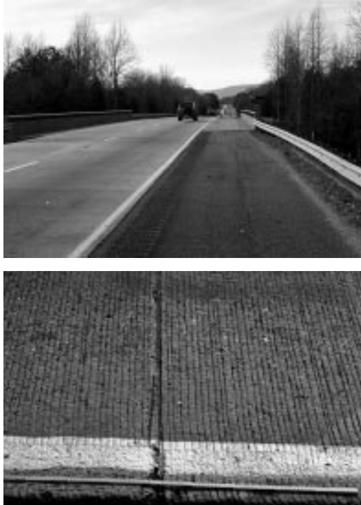
FIGURE 2 Interstate 64's continuously reinforced concrete pavement, reconstructed in 1987, near Charlottesville, Virginia, after 14 years of service. Pavement is in excellent condition, as shown in lower photo.
