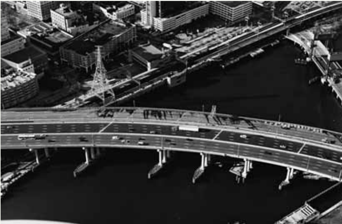
Interstate-95 in Bridgeport, Connecticut, is undergoing reconstruction to repair aging infrastructure.
