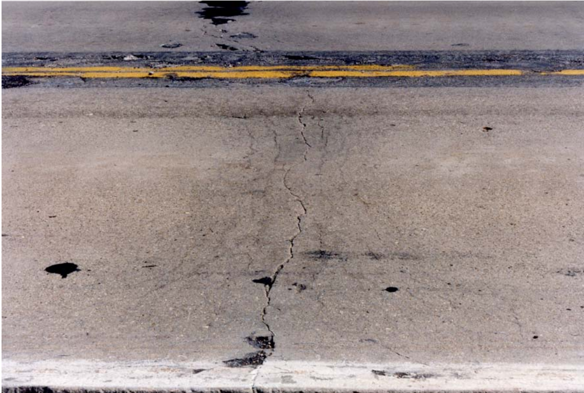
FIGURE 2 D cracking distress at transverse crack.
