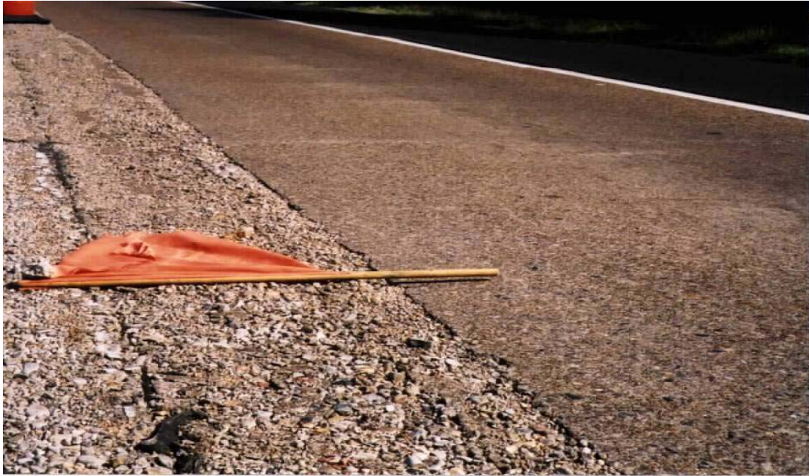
FIGURE 3 Vertical displacement prior to rolling.
