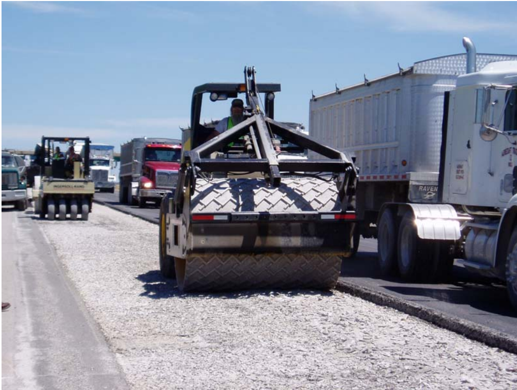
FIGURE 4 Z-pattern steel grid roller.
