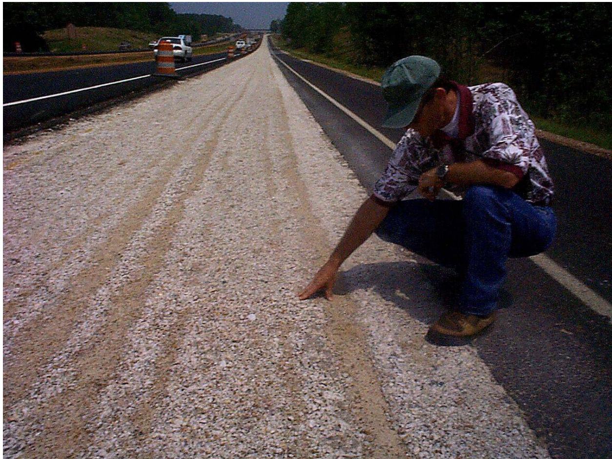
FIGURE 7 Resonant rubbleized PCC, before rolling.
