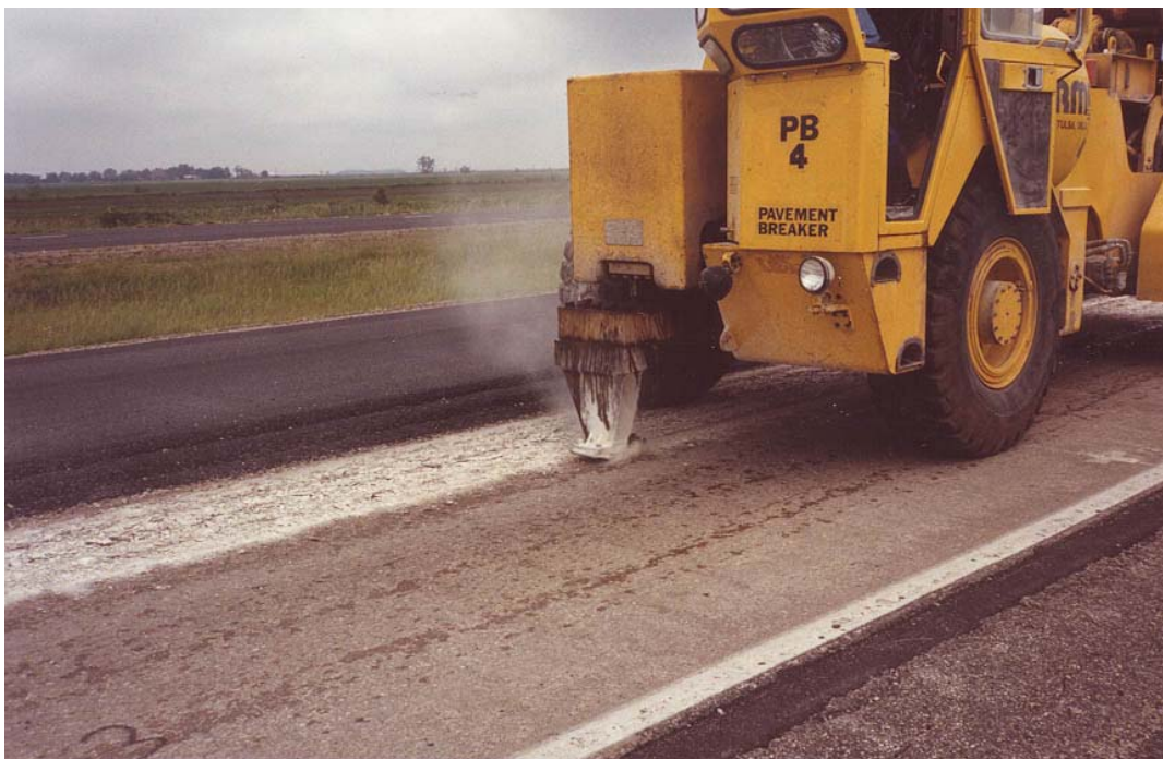
FIGURE 5 Resonant frequency breaker.
