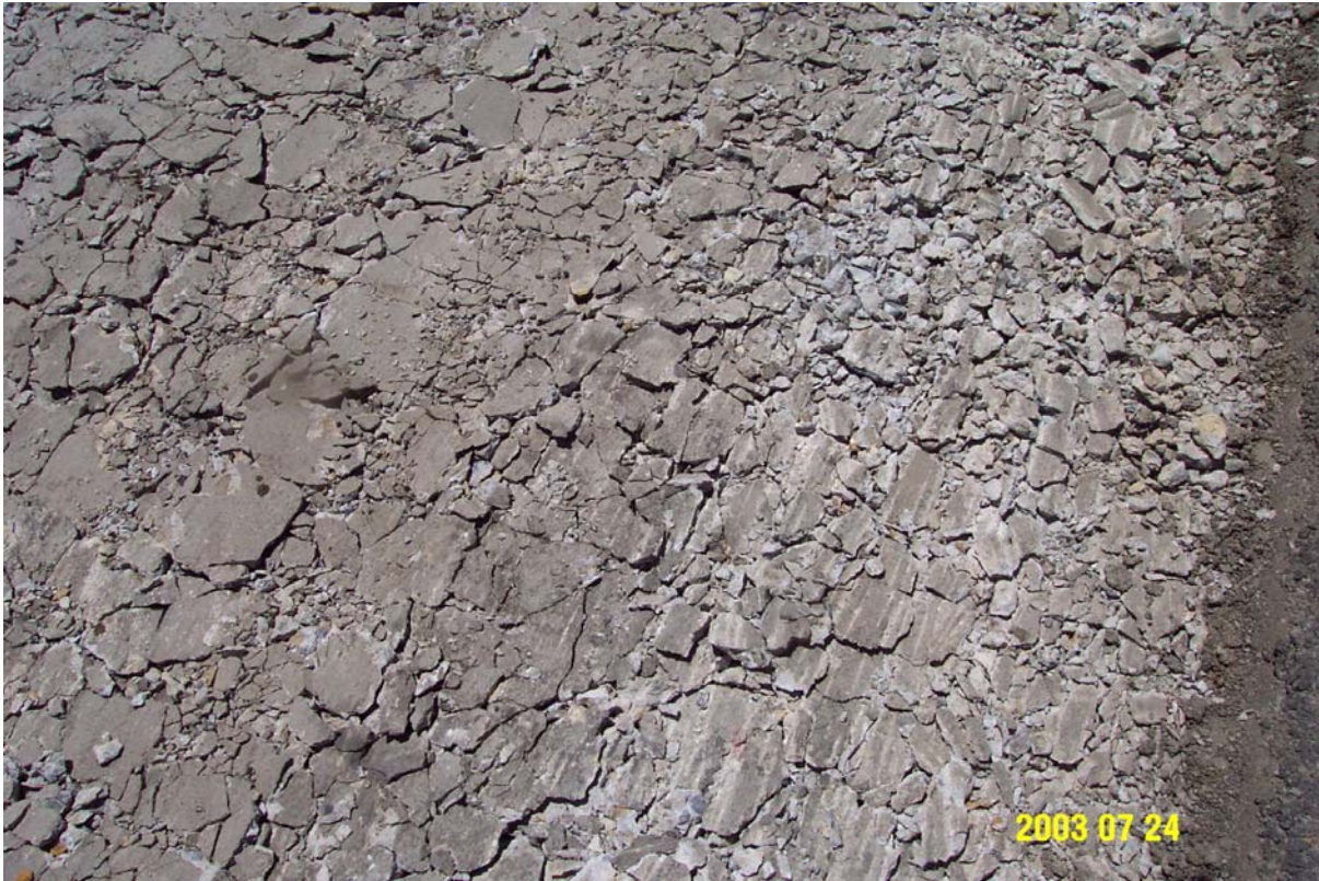
FIGURE 5 Note the “flaky” rubblized PCC surface.
