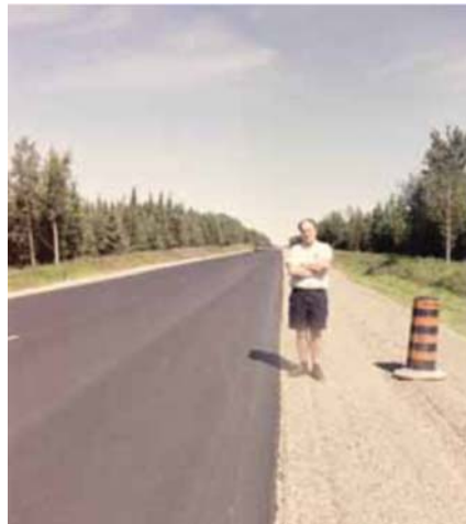
Highway 655 pavement test site in northern Ontario just after construction and apparently before the cold spell
