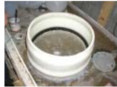
10-inch section of 12- inch diameter PVC pipe
