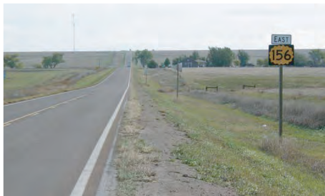
Before improvements were made along K-156, a sloping dirt shoulder didn't allow motorists adequate room to pull off of the highway.
