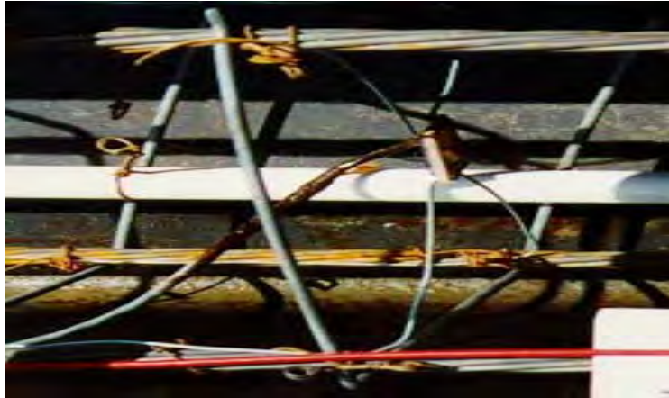
(a) Typical Sensor Installation
