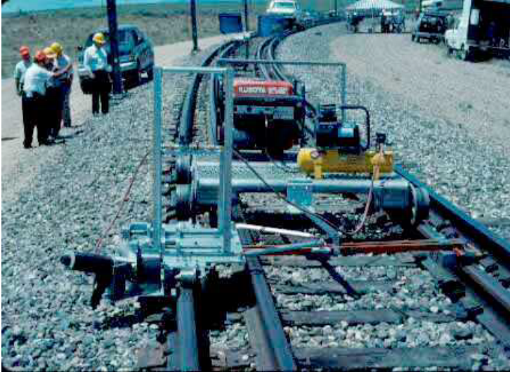
Figure 1 Cart for application of optical fiber to rail
