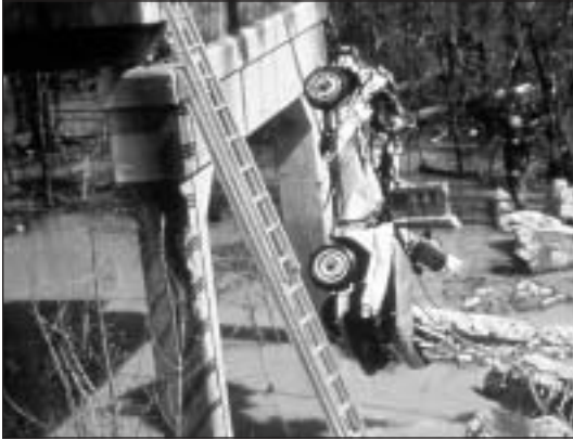
FIGURE 1 Failure of a bridge pier as a result of channel migration led to collapse of bridge over the Hatchie River, Tennessee, in 1989.
